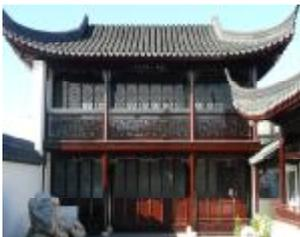
The method of laying the tiles followed traditional tiling techniques from China and they were placed by artisans with special skills in this field of work. The curve of the rooves is traditional and each tile is overlaid by the next one by 80%. The sweeping corner ridges on each structure were created by one particular artisan who was also responsible for the
