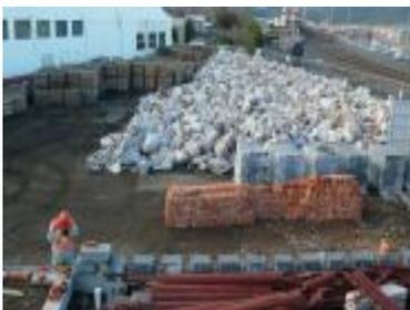
Approximately 1000 tonnes of rock were transported from the quarry at Lake Tai coming in over in 50 containers. Over 2/3<sup>rd</sup> of the rock was used to create the artificial hill the design of which is very much in the mind of the particular artisan who has the expertise in the design of such features The balance of the rock was used to line the edges of the pond and to create the rock features in various parts of the garden.
