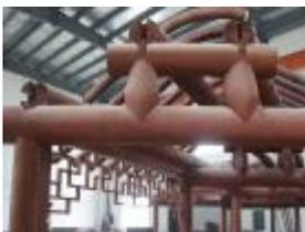
The extensive timber frameworks in the structures are very flexible and absorb the energy in an earthquake by deflection within the framework. All the jointing is by mortar and tenon with wedges so the whole is intimately bound together. The base of the timber columns are held in position by the walls
