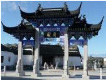
The four granite columns, which support the structure and are on average 5-6 m long, were all excavated as four whole single columns something which is unusual today. The form follows traditional Chinese design with the sweep of the ridges matching those in the buildings with the Garden and which are very much the signature of an individual artisan.
