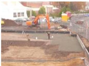
Retention of the water in the pond and separation of the pond water and groundwater is provided by way of a geosynthetic membrane (essentially a layer of bentonite retained between two synthetic fabric layers) which is protected by layers of specially selected gravel above and below the membrane and which is laid under the whole of the garden. It is “self-healing” by which is meant that if it is penetrated in any way it will quickly seal again owing to the presence of the bentonite.
