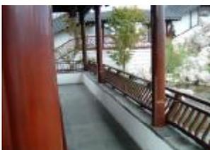
Low walls topped with a ceramic slab and a vertically curved timber balustrade provides seating in some areas (such as the pavilion in the pond, around the Main Hall exterior corridor and in the Entrance Hall). Such curved seating is known as the “slumbering woman” seating.
